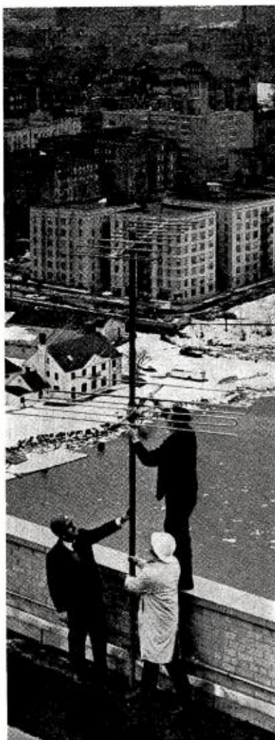
High above the Harlem River, workers for CATV Enterprises align an antenna at the head-end site atop a 28-story apartment building.
